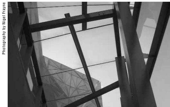
View from the eastern atrium stairwell, ACMI, Federation Square, Melbourne
