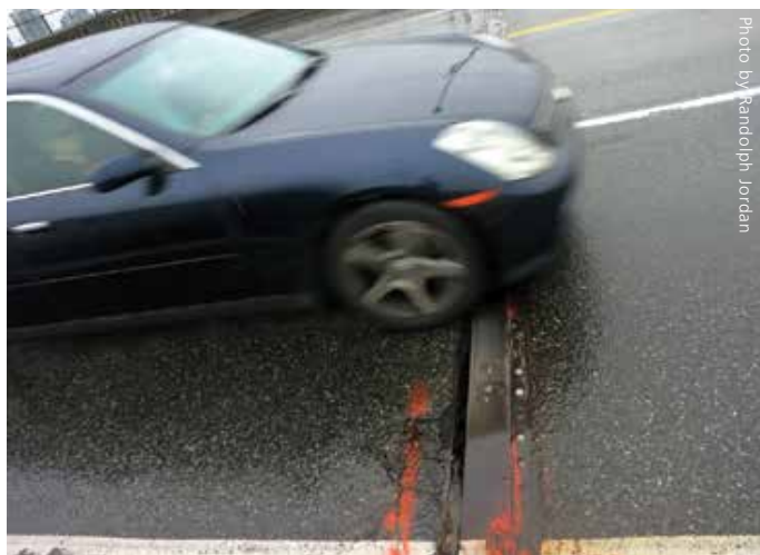
Fig. 1. (Left) Archival photo of Vancouver's Burrard Bridge, 1936. Fig. 2. (Above) Pothole atop of the southwest concrete pillar
