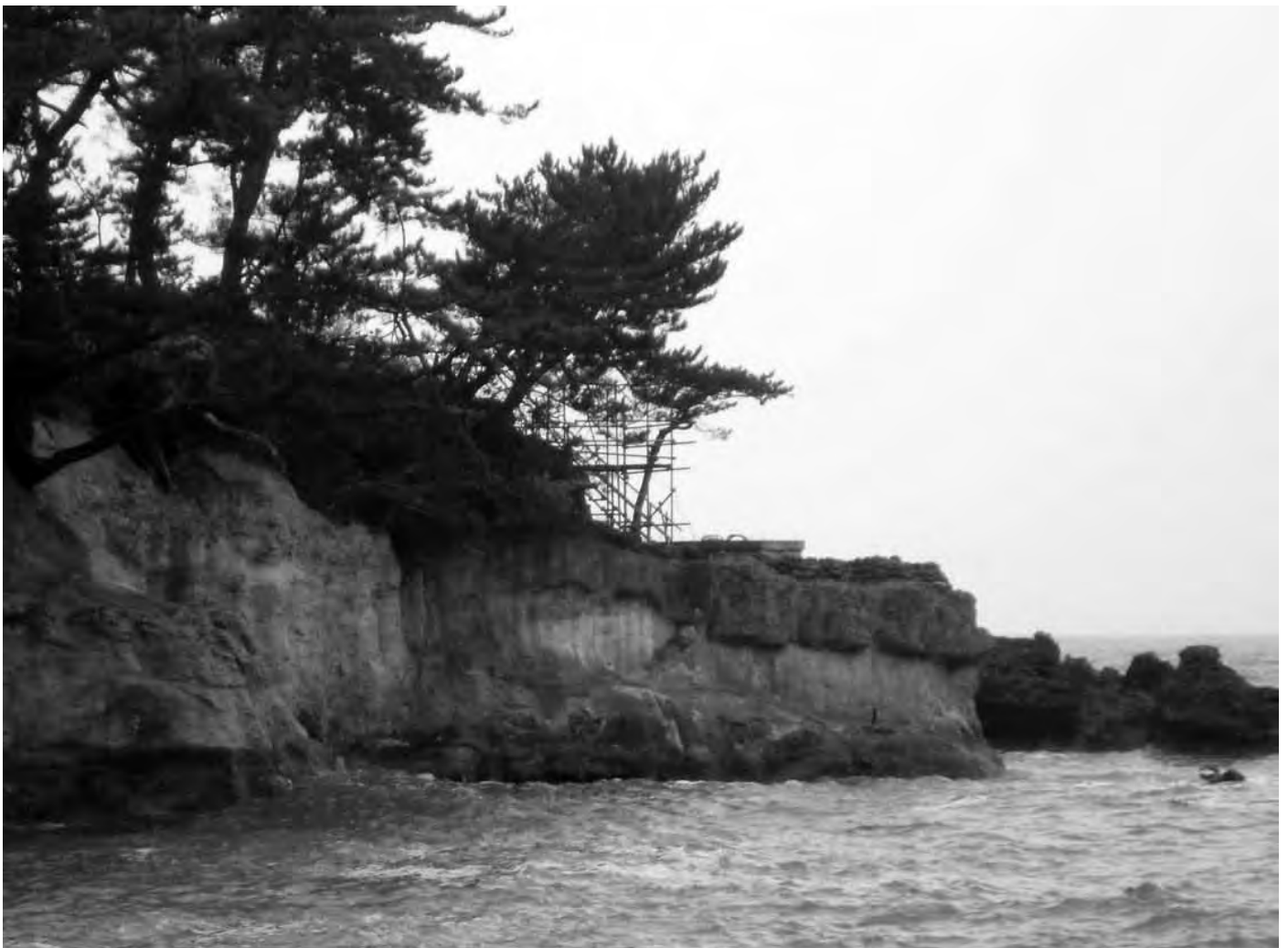
Fig. 7: The site and the surroundings of the pavilion after it was swept away by the first wave, leaving only its base . Photo by Keiko Torigo
